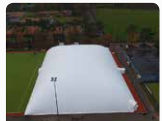
RSI double membrane installation: HOD Valkenswaard
